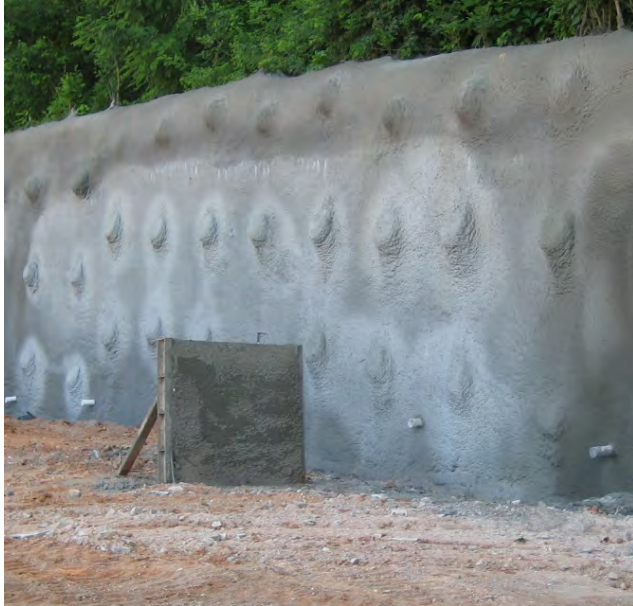
Figure 3.10: Photo. Curing of a shotcrete test panel on site. Photograph courtesy of Schnabel Engineering.
