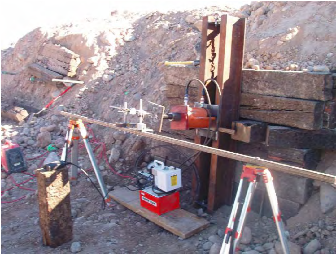
Figure 9.1: Photo. Soil nail load testing setup. Source: Cadden et al. (2010).
