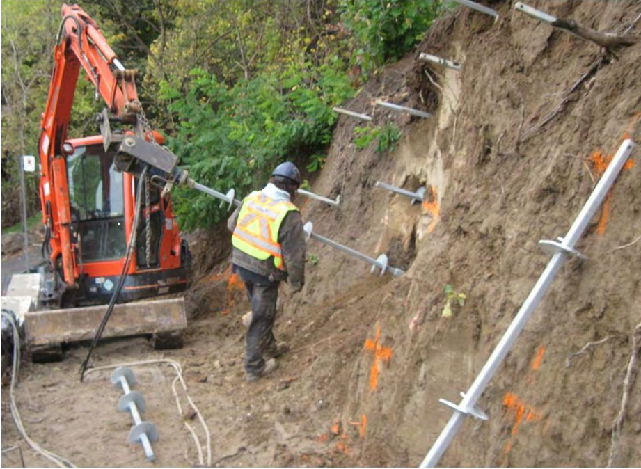
Figure G.2: Photo. Screw-in nail installation. Photograph courtesy of Hubbell Power Systems, Inc.
