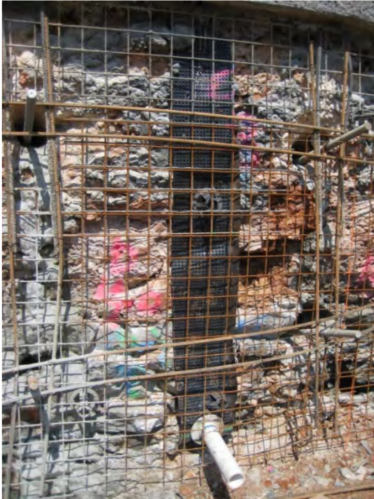
Figure 3.12: Photo. Strip drain prior to initial shotcrete placement. Photograph courtesy of Schnabel Engineering.
