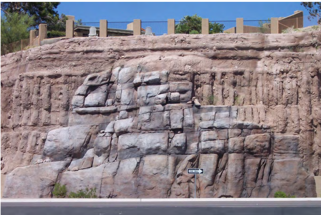
Figure 3.22: Photo. Sculpted natural rock-like wall facing. Photograph courtesy of Con-Tech Systems, Ltd.
