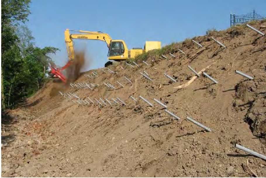
Figure G.1: Photo. Launched nail installation. Photograph courtesy of GeoStabilization International.
