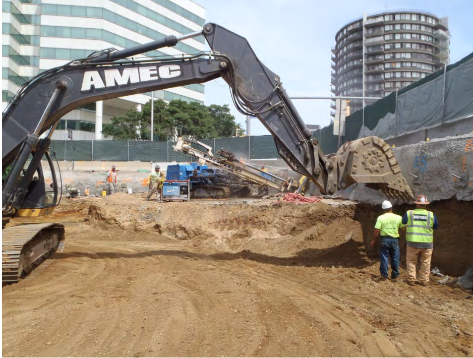
Figure 3.13: Photo. Excavation of soil lift during construction of soil nail wall. Photograph courtesy of Moretrench American Corporation.
