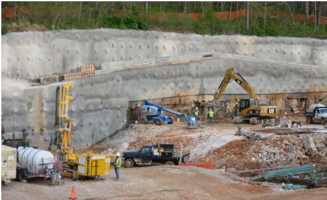
Figure 2.3: Photo. Construction of soil nail wall. Photograph courtesy of Schnabel Engineering.
