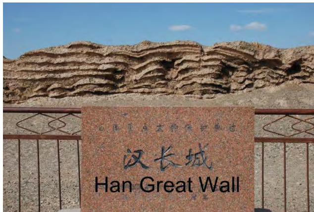
Figure 10.1 The Han Great Wall (photo courtesy of Xue).
