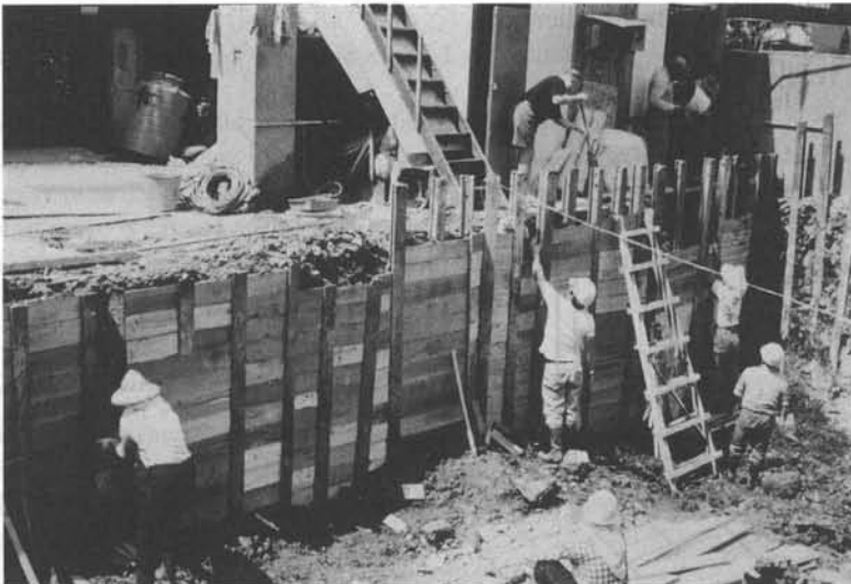
Figure 3.16 Photo of the soldier pile method.
