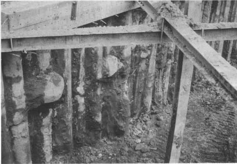
Figure 3.20 Photo of column piles.
