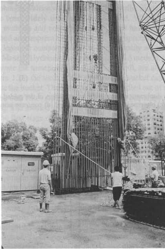
Figure 3.28 Photo of the diaphragm wall method.
