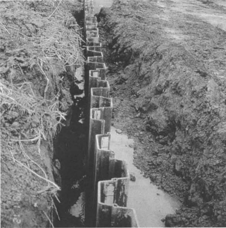
Figure 3.18 Photo of the steel sheet pile method.
