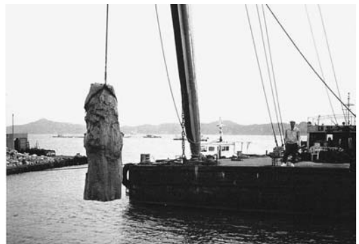
FIGURE 2.17 Grout mass resulting from underwater injection.
