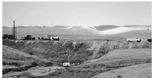
FIGURE 11.25 Typical embankment on the California Aqueduct.
