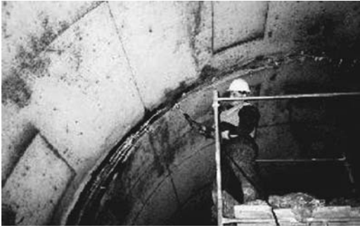
FIGURE 17.11 Open joint was caulked to minimize leakage during injection.
