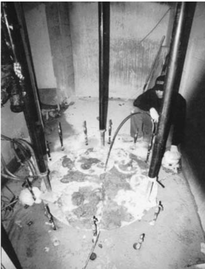
FIGURE 20.9 Grout injection around a sand-filled and shored open-top tank.
