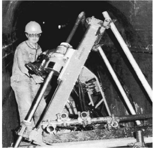
FIGURE 30.1 Power feeds with hollow chucks are used in confined areas.
