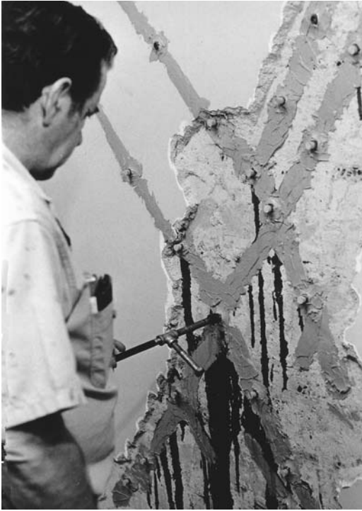
FIGURE 1.1 Epoxy injection to repair cracks in concrete.
