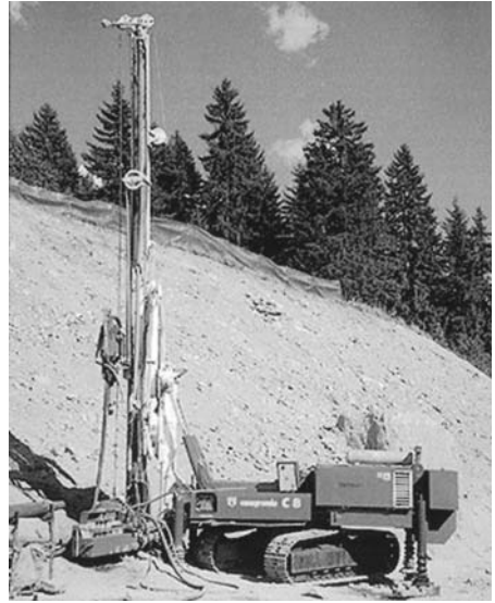
FIGURE 30.7 Large powerful self-contained hydraulic drill rig for large or deep holes.
