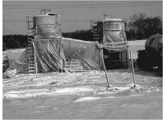
FIGURE 18.4 Shelter built around grout plants and material supply.
