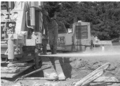
FIGURE 2.27 High-pressure jet for one-fluid jet grouting system.
