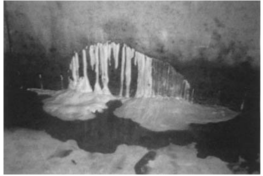
FIGURE 17.9 Return of polyurethane grouts is plainly visible.
