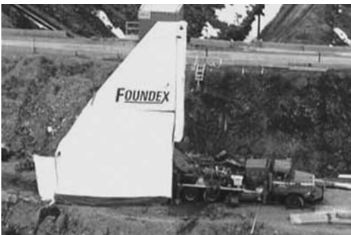
FIGURE 18.5 Special enclosure attached to drill mast to protect the drilling operation.
