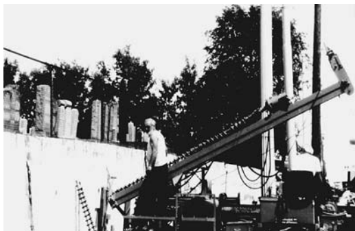
FIGURE 19.11 Augering of tieback holes.
