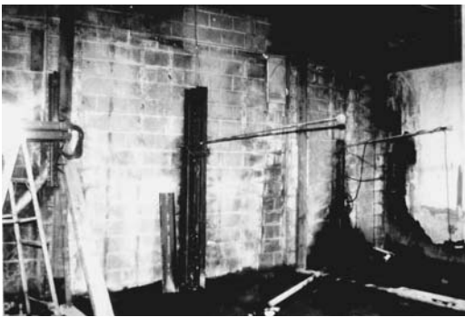
FIGURE 19.13 Tie-back rods provide restraint for whaler system.
