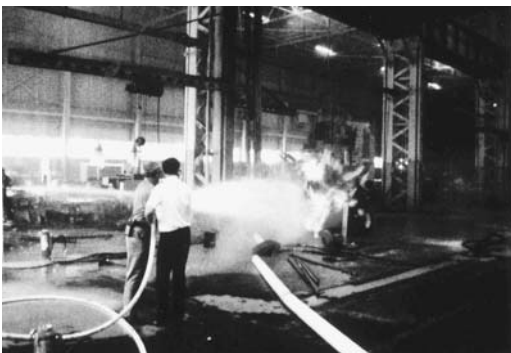
FIGURE 19.17 Adjacent column can be seen as the fire is extinguished.
