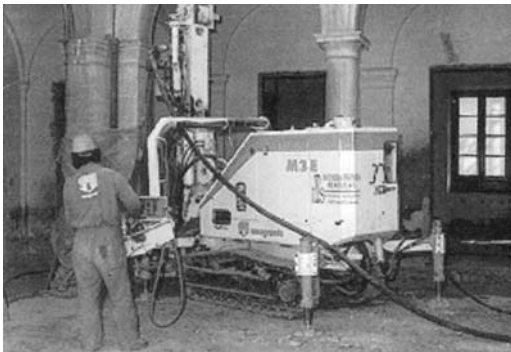
FIGURE 30.6 Small self-contained hydraulic drill rig inside a building.
