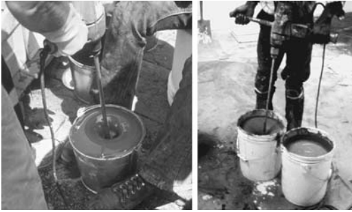
FIGURE 33.1 Jiffy mixer blending resin in small container (left) and larger paddle mixer preparing 5-gal batches (right).
