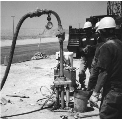
FIGURE 2.21 Extraction jacks and proprietary casing with grout header and wide-sweep bends.
