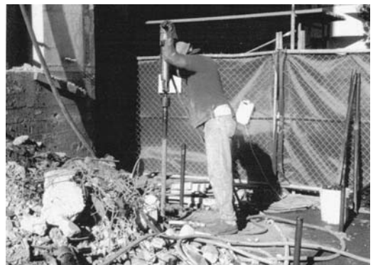
FIGURE 10.27 Standard pneumatic hammer used for driving casing.
