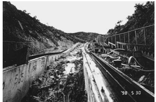
FIGURE 12.15 Tracks placed on continuous guide walls up a dam abutment slope.
