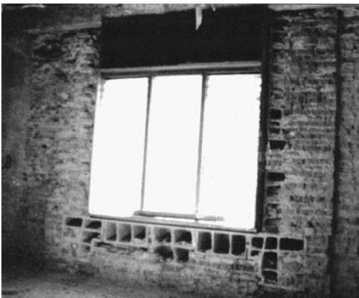
FIGURE 2.4 Large unfilled cells are typical of older terra-cotta masonry cladding.
