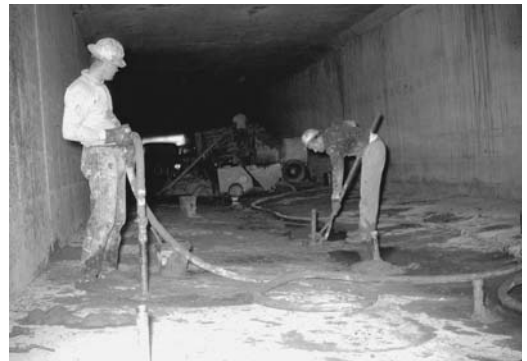
FIGURE 38.2 A culvert raised to the proper grade.
