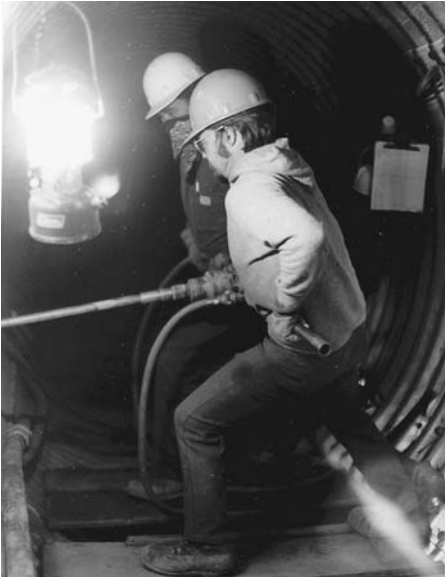
FIGURE 15.4 Space limitations usually require compact drills and short drill rod sections.
