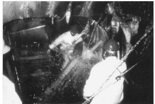
FIGURE 17.16 Core drilling in dam gallery.
