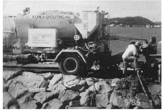
FIGURE 11.39 The grout plant located on an adjoining jetty.
