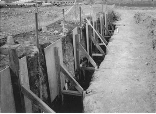
FIGURE 2.9 Test site excavation to allow visual inspection of grout masses.
