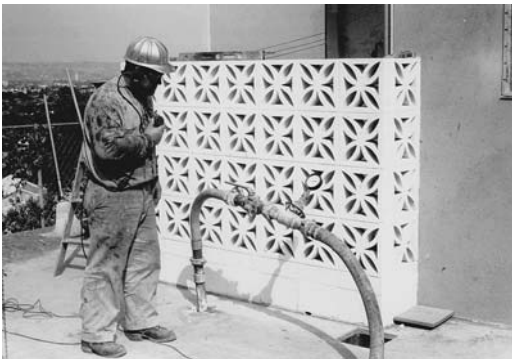
FIGURE 11.7 Wide-sweep bend and full-diameter fittings used in compaction grouting.
