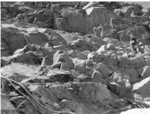
FIGURE 12.11 Very rough finished surfaces are common with some rock types.
