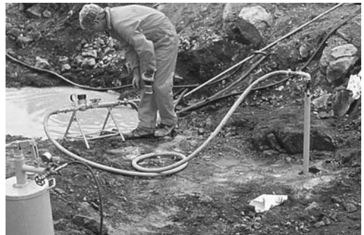
FIGURE 12.2 Typical water test in progress.
