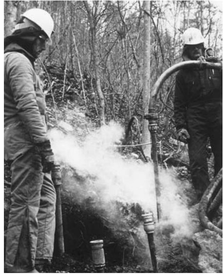
FIGURE 20.11 Smoke rising from the ground as the grout is injected.
