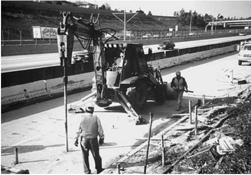
FIGURE 11.20 A hydraulic casing driver mounted on a standard backhoe.
