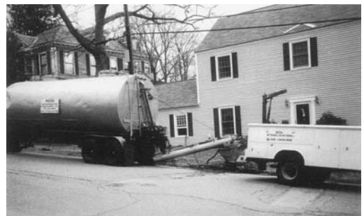
FIGURE 33.5 Contractor-built bulk material handling, proportioning, and pumping setup.
