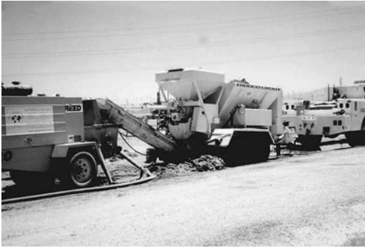
FIGURE 28.2 Equipment and worksite were kept clean and orderly.
