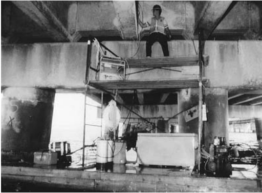
FIGURE 7.16 A household chest freezer is used to cool epoxy components in warm weather.
