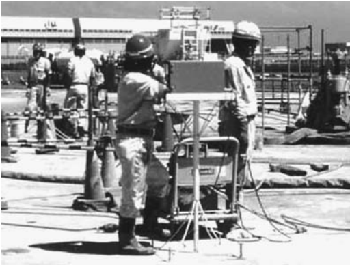
FIGURE 11.24 Data are transmitted to a pump from a portable control station.
