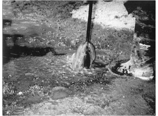
FIGURE 10.38 Flushing a grout hole until only clear fluid returns.
