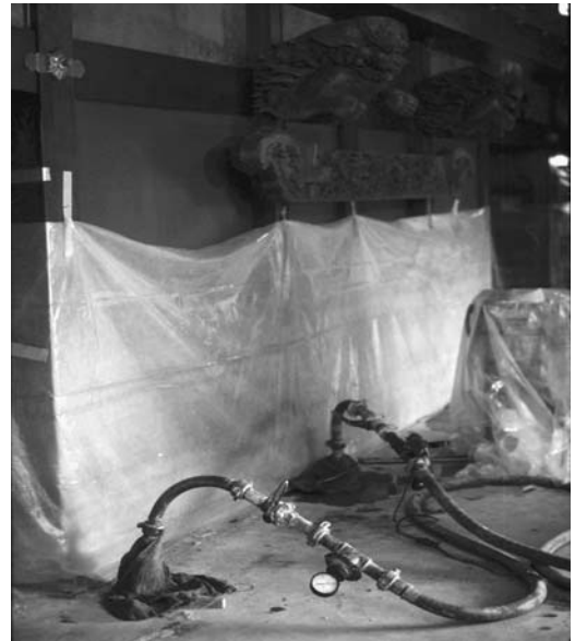
FIGURE 20.10 Emergency slabjacking in progress. Note protection on decorative wall.
