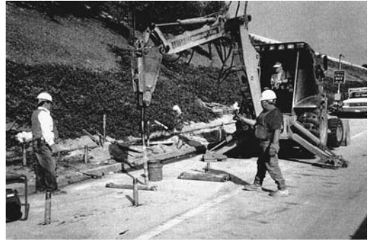
FIGURE 10.26 Large equipment-mounted hydraulic driver.
