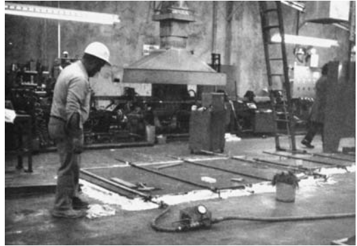
FIGURE 1.5 Structural grouts are injected to provide support to base plates.
