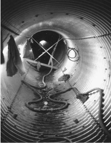
FIGURE 15.9 The overhead holes were the last grouted.
