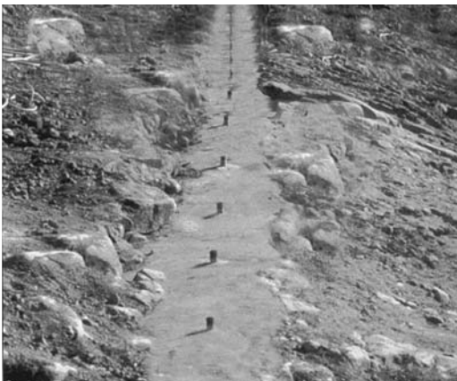
FIGURE 10.35 Standpipes are sometimes embedded in a concrete grout cap.
