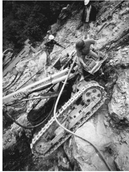
FIGURE 30.10 Relatively light weight and low center of gravity allow air tracks to be literally hung.
