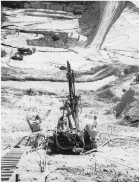
FIGURE 30.9 Air track held on steep abutment slope with a winch.
