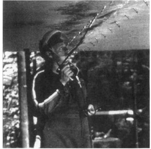
FIGURE 17.10 Angled holes intersect the interior of joint.
