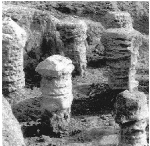
FIGURE 2.26 Exposed columns of soilcrete resulting from jet grouting.
