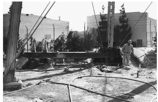
FIGURE 20.8 Emergency shoring and a tent erected to preclude flooding while grouting.
