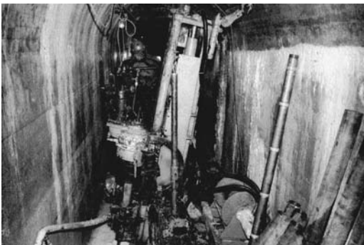
FIGURE 10.17 A powerful independently powered hydraulic drill fills this dam gallery.
