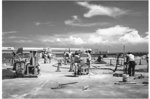
FIGURE 11.23 Compaction grouting under active runways and taxiways.
