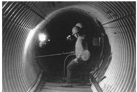
FIGURE 10.20 Drilling in a culvert with a handheld pneumatically powered drill.
