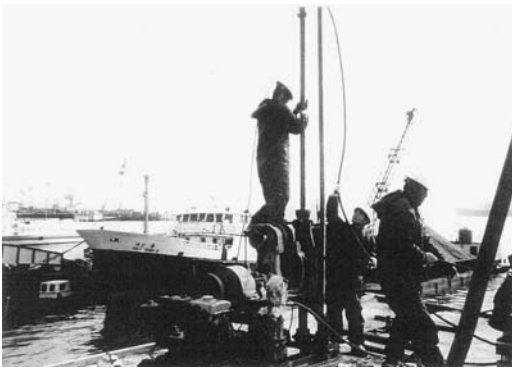
FIGURE 11.38 Drilling an underwater hole from a pier.
