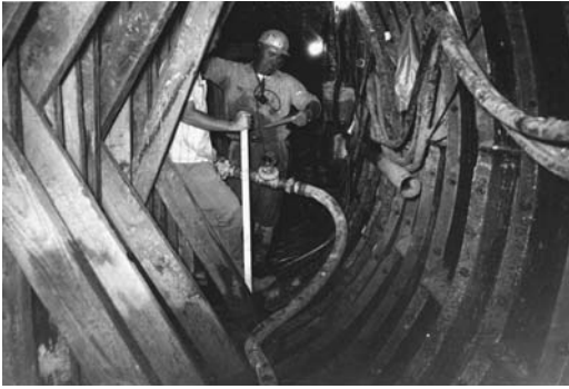
FIGURE 15.7 Vertical shoring is often required when lifting large conduits.
