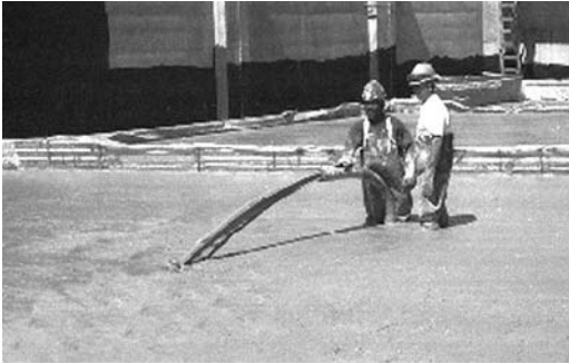
FIGURE 5.15 CLSM grouts can be nearly self-leveling.
