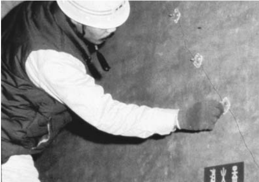
FIGURE 10.1 Surface-set injection port over a crack.
