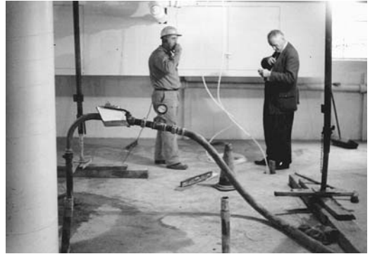
FIGURE 11.21 Piezometer tubes hanging from the ceiling indicate pore pressures greater than the overburden pressure.
