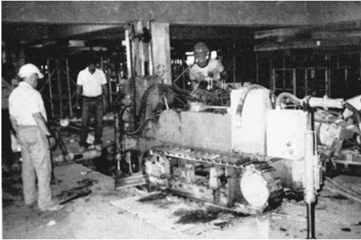
FIGURE 10.14 Self-contained fully hydraulic drill rig.
