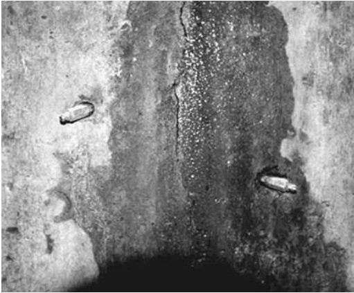
FIGURE 17.3 Typical staggered holes angled to intersect the defect.
