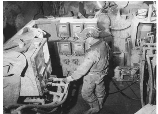
FIGURE 9.13 Computer monitoring equipment at the grout plant allows the operator immediate observation of the injection parameters, facilitating prompt adjustment.
