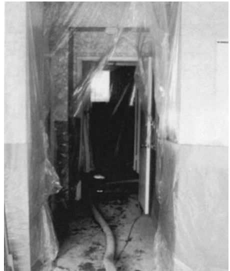
FIGURE 11.43 The walls were protected with plastic sheeting.
