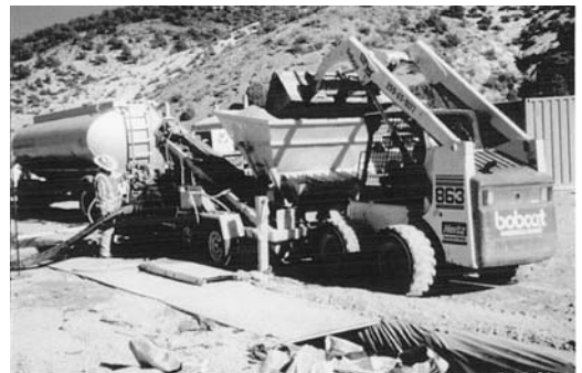
FIGURE 11.50 Mixer supplied with aggregate by a skid steer loader.
