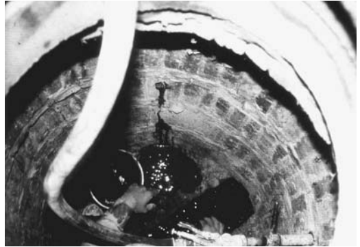
FIGURE 17.12 A cement-filled acrylic grout integrated poorly bonded brick.
