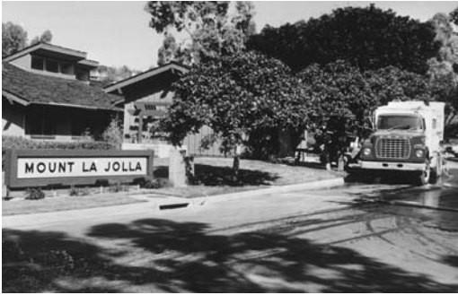
FIGURE 11.42 Severe settlement occurred in many buildings in the Mount La Jolla development.
