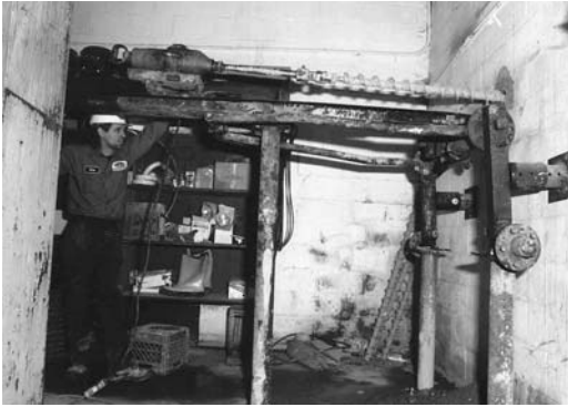
FIGURE 19.12 An especially fabricated drill rig was used for drilling anchor holes.
