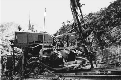
FIGURE 12.16 Powerful drill rig is able to operate from rail-wheel-mounted platform.
