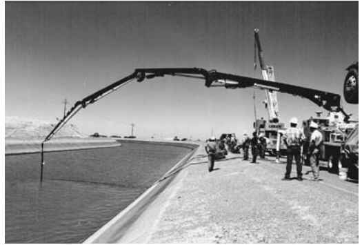
FIGURE 20.6 Ready mixed grout was rapidly pumped to stop leakage.
