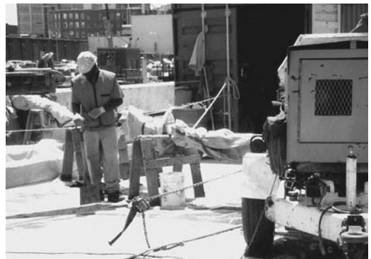
FIGURE 18.1 Insulation of the grout delivery line to prevent excessive heating.
