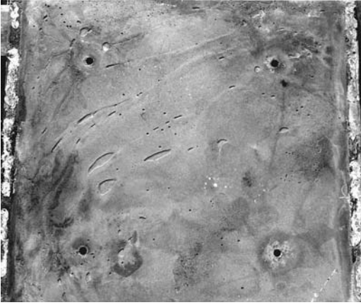
FIGURE 6.9 Top plates removed to allow visual inspection of any remaining voids.
