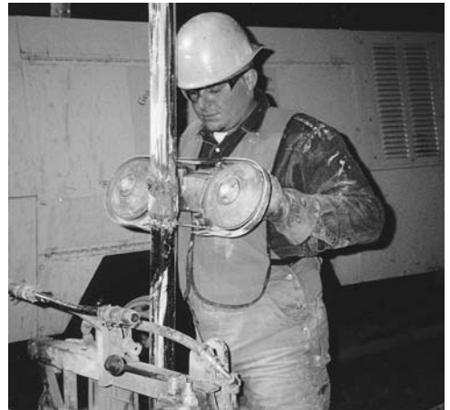
FIGURE 11.4 Casing with welded joints during placement will require physical cutting during withdrawal.
