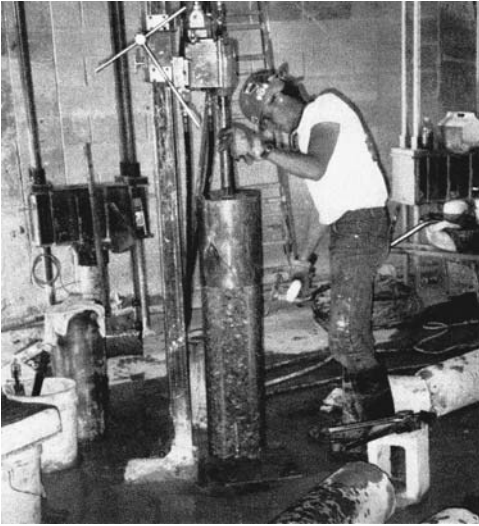
FIGURE 10.25 Highly portable drills are temporarily anchored to surface being drilled.
