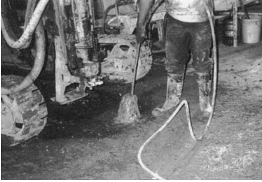
FIGURE 12.3 Washing out the hole to thoroughly clean it of all cuttings or other deleterious matter.
