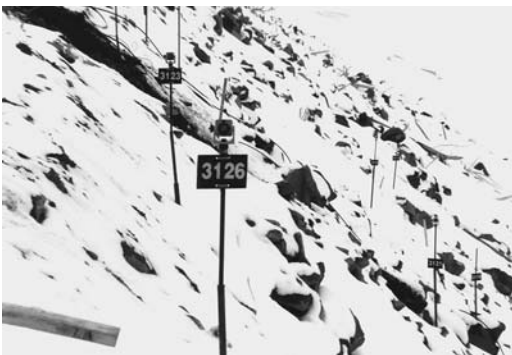
FIGURE 11.34 Arrays of prisms were constantly scanned to detect any surface movement.
