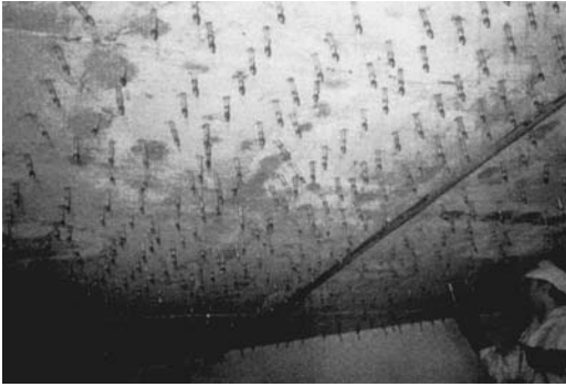
FIGURE 17.5 Porous areas will require a grid of closely spaced ports.
