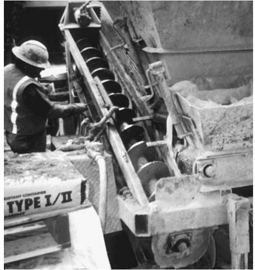
FIGURE 33.6 Typical auger mixer for low-mobility grouts.
