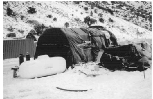
FIGURE 18.9 Water tank insulated with heavy concrete curing blankets.
