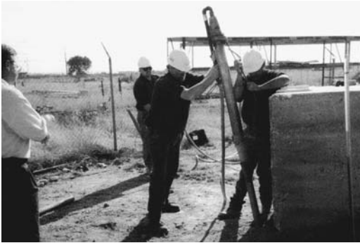
FIGURE 10.28 Pipe rammers provide high-energy, low-frequency pounding.
