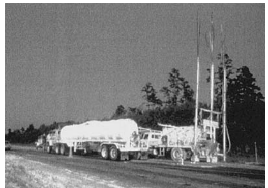
FIGURE 2.25 Multiprobe lime injection rig.
