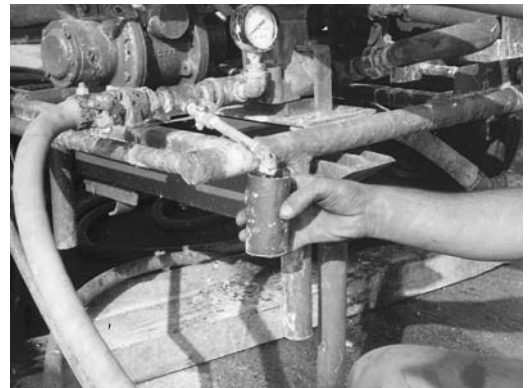
FIGURE 4.9 A sampling valve facilitates the gathering of set time specimens.
