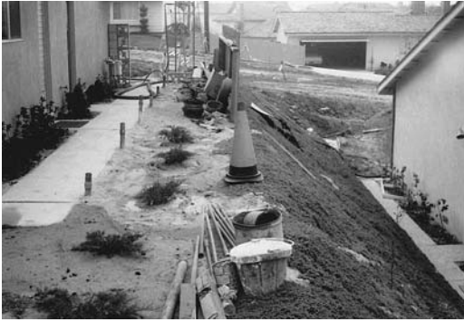
FIGURE 11.40 Row of grout holes (left) adjacent to typical compacted fill downslope.
