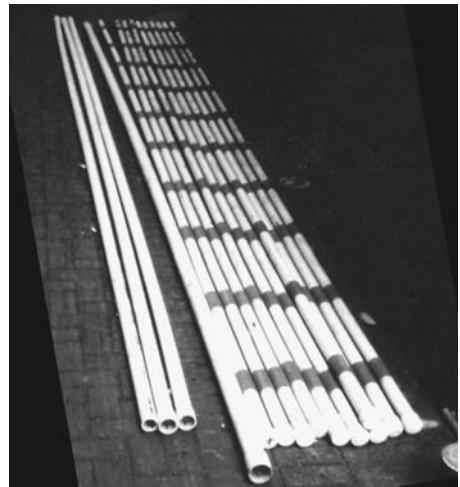
FIGURE 30.23 Sleeve port pipe awaiting installation, solid pieces on left are for nongrouted zone.
