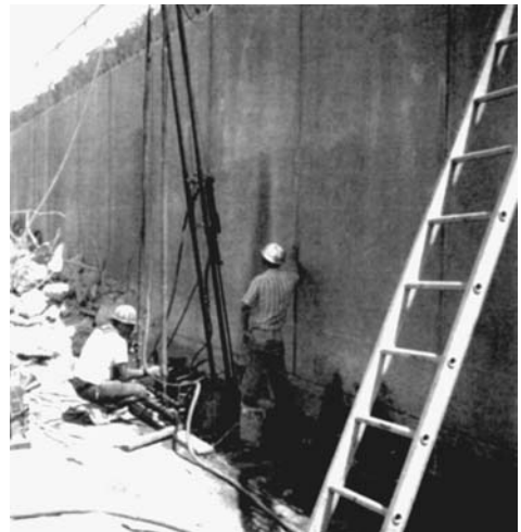
FIGURE 10.29 Light frame with winch for handling drive needles.
