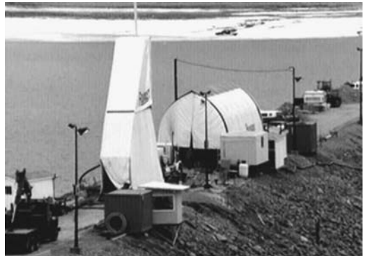
FIGURE 11.32 Heated shelters were required to withstand the cold winter conditions.
