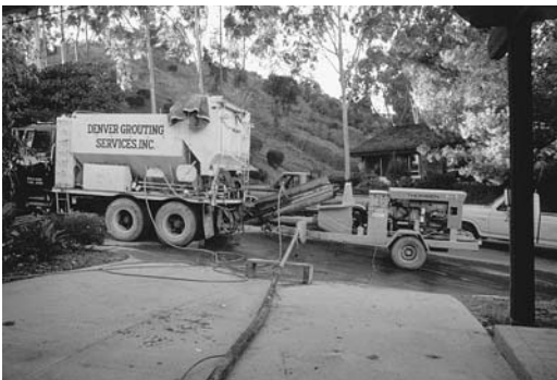
FIGURE 11.45 The mixing plant and pump remained on the fronting street.
